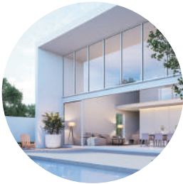
Whole-house water treatment
